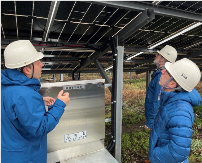
Glennmont on site with correct PPE
