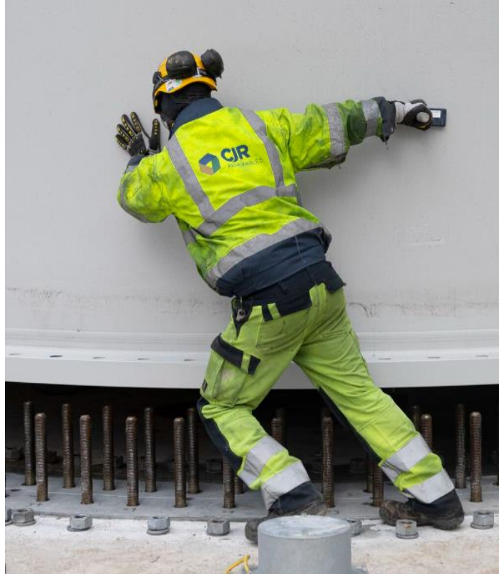
1 Solar PV Plant Construction Site 2022 2 Onshore Wind Plant Construction Site, 2022
